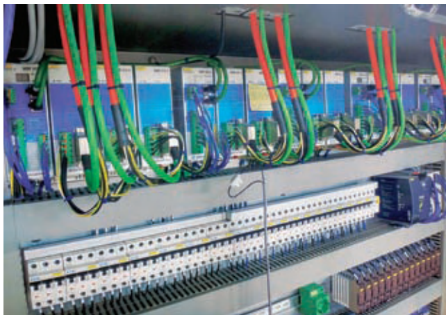
For precise control of the servo motors, the modular multi-axis servo system »Dias-Drive MDD 100« is used.
