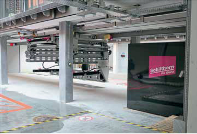
The process of docking a container to the cable car cabin.
