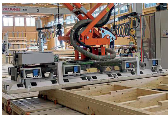
The position has been reached, and the insulation material is being blown in.
