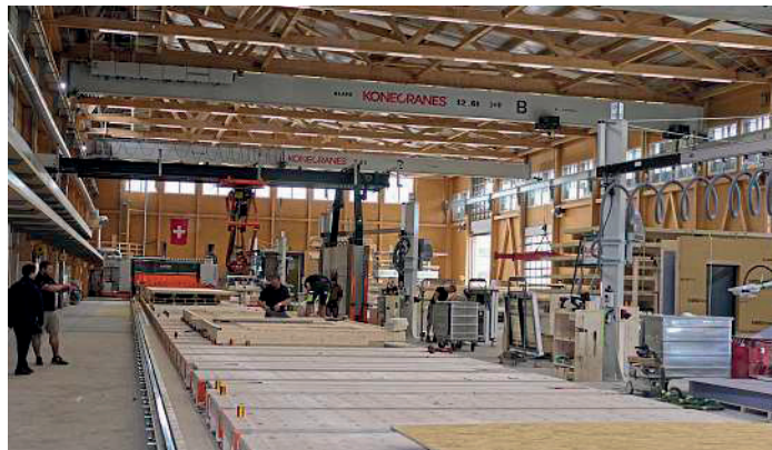
Work preparation for the blow-in process.
